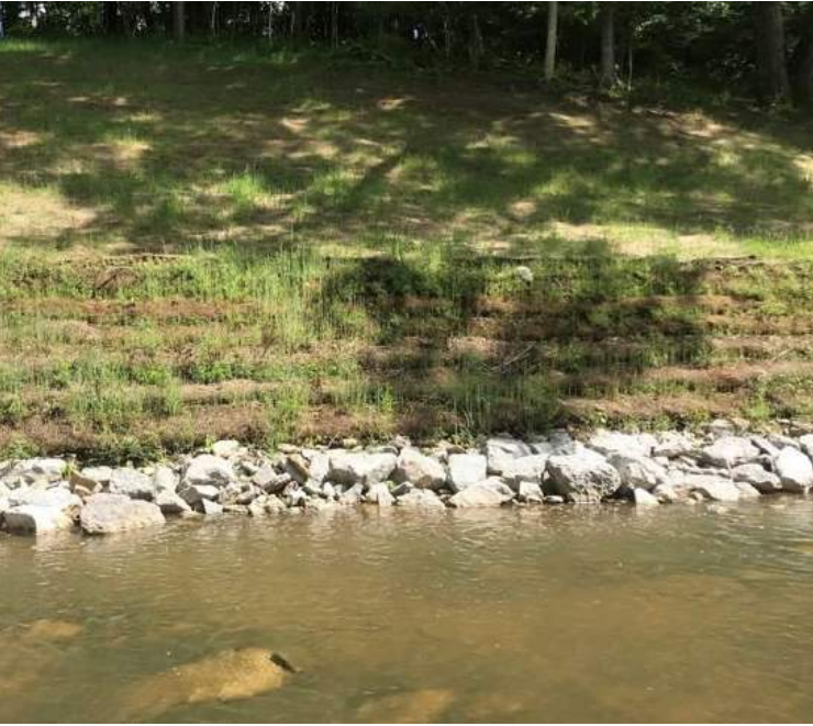
Picture taken 1-month post-construction
