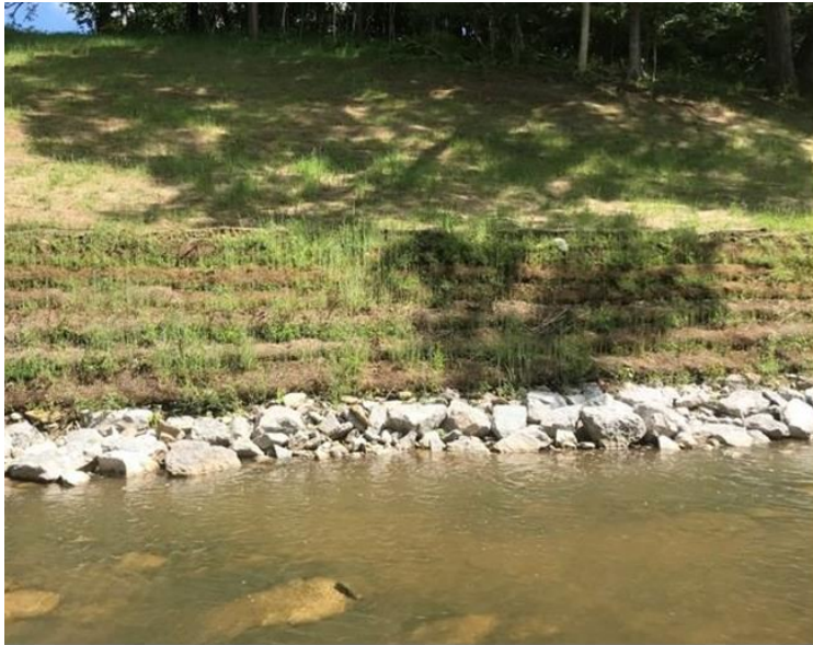
Picture taken 1-month post-construction
