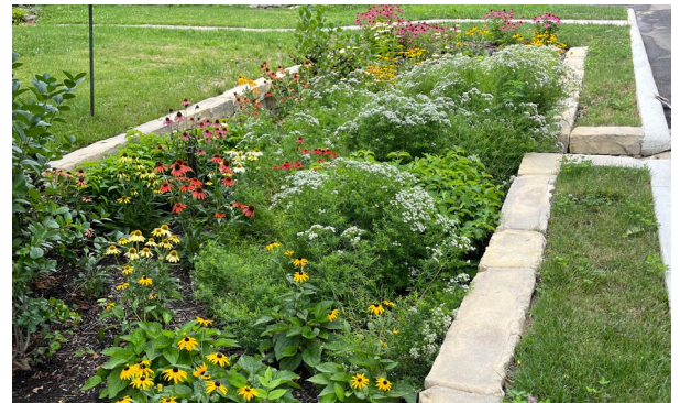
Completed basin in North Linden 1
