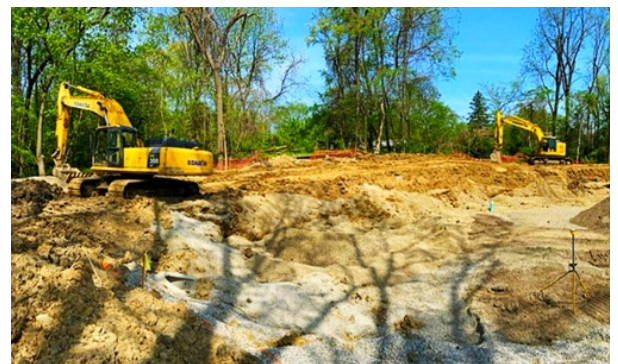
Construction underway in Linview Park
