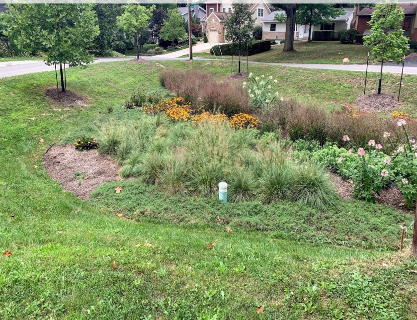
Regional rain garden
