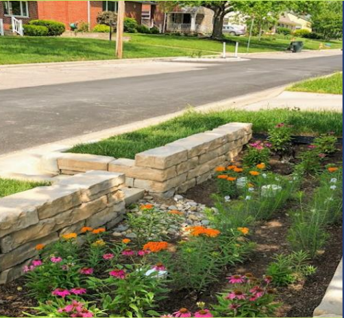
Behind-the-curb rain garden- 2 walls
