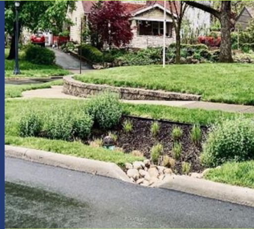
Behind-the-curb rain garden- no walls
